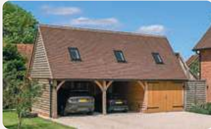
3 bay Gloucester with larch weatherboarding and joinery
