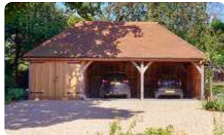
3 bay Canterbury with oak weatherboarding and joinery
