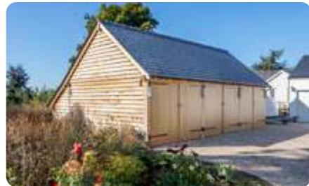
3 bay Canterbury with oak weatherboarding and joinery
