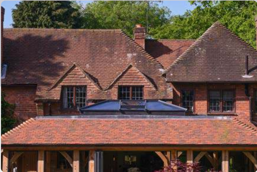
Opposite: Oak rafters in the extension roof continue the traditional style of the home into the newly created dining room. Above right: The lantern sits over the dining table and is surrounded by spotlights. Above left: The mansard roof allows views from the bedrooms and the tiles are matched perfectly with the existing roof.
