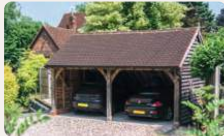
2 bay Kenchester with oak weatherboarding
