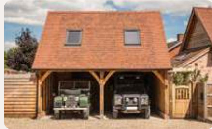
2 bay Little Gloucester with oak weatherboarding
