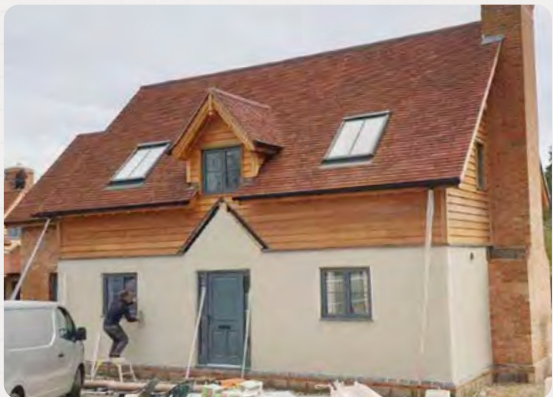
6. Your home is nearly complete ready for Building Control sign off, access through all your doors with hard landscaping will be required.
