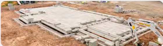
1. Ground workers will prepare the foundations for your home with pads for the oak posts and perimeter blockwork for the wall panels. Your oak frame and wall and roof system will be being prefabricated in our workshops at the same time.
