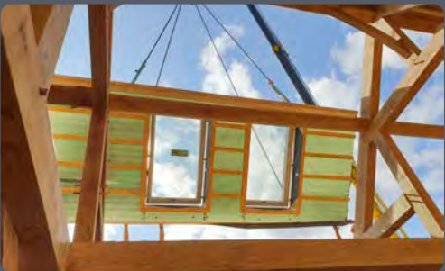
2. Your dedicated Oakwrights project manager will check the site is ready for the oak frame and wall panels. Progress will be made quickly with the frame, then the pre-insulated wall and roof system will be installed in a matter of weeks using a crane. Take your project further with our Posi-Joist floor.
