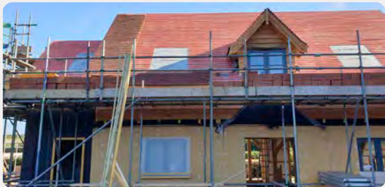
3. Achieving dry shell status, a weatherproof shell will mean you can commence all the interior work. Oakwrights can supply and install windows and face glazing will be installed last of all. If you are choosing to sandblast your oak frame, do it now.
