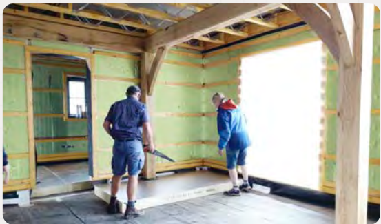
4. The first fix stage includes many trades all installing the hidden parts of your water, heating, electrics and ventilation and more insulation. Time to book your AeroBarrier install to achieve first class airtightness.
