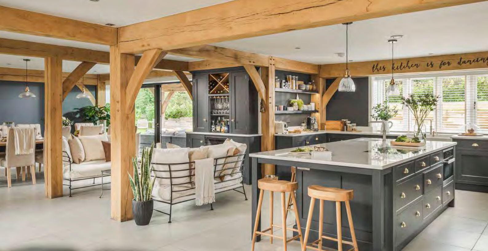
The open-plan ground floor features zones clearly defined by the oak post and beam frame, with the full bay kitchen and dining areas flanking a half bay seating area.
